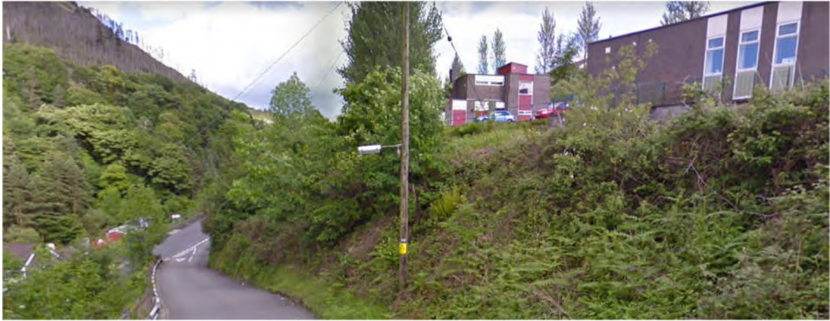
EXISTING CYMMWR HEALTH CENTRE VIEWED FROM CYMMWR VIADUCT
