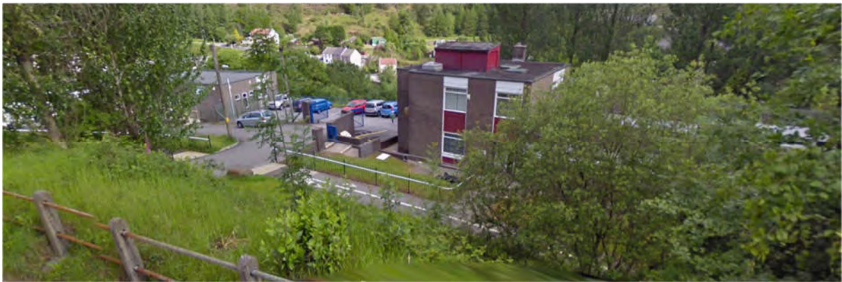
EXISTING CYMMWR HEALTH CENTRE VIEWED FROM STATION ROAD
